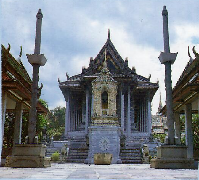
Front view of the Ordination Hall of Phra Phuttha Rattanasathan. A pair of pavilions and stone pillars for lantern hanging on both sides. In the middle stands a Mondop-spire belfry adorned with Chinese ceramic.
